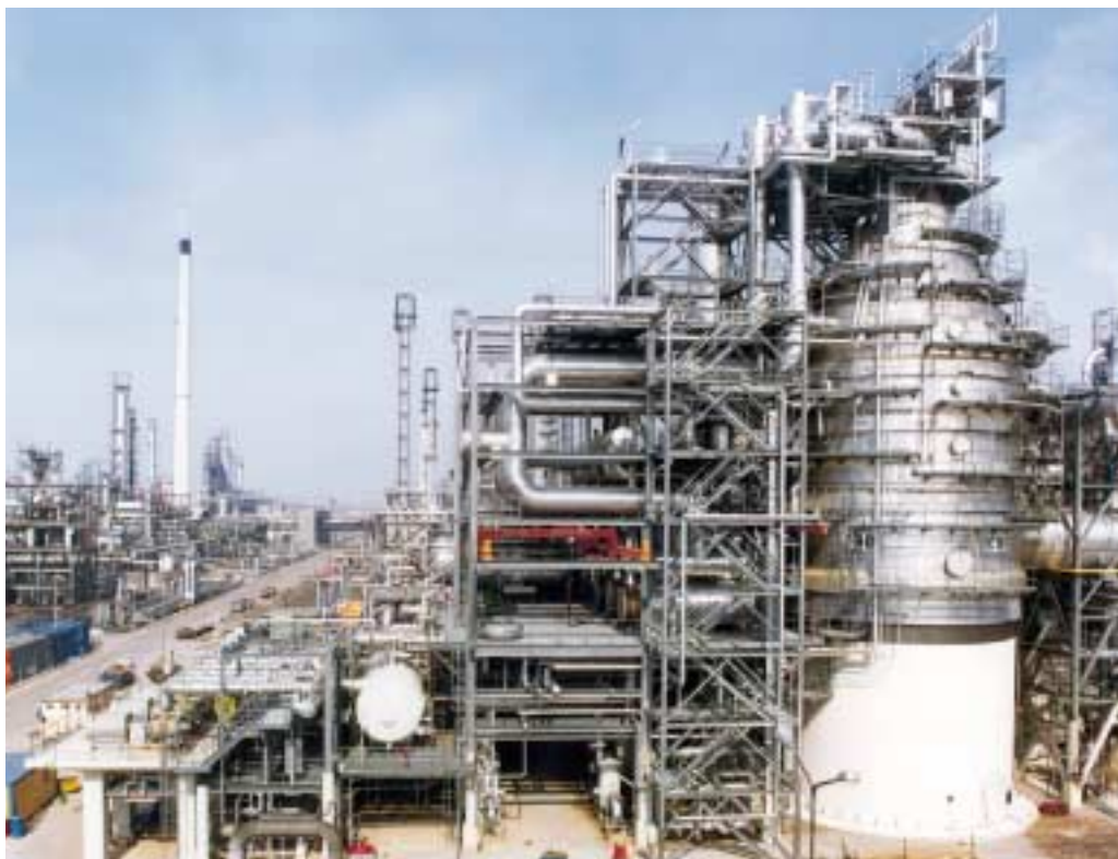
Steam jet liquid ring vacuum pump for the distillation column of a refinery
